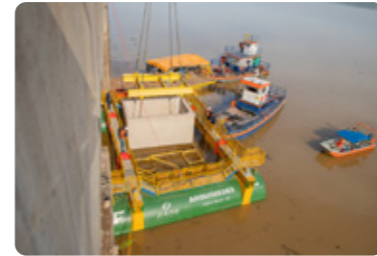
Deployment of structures for anchoring the floats.
