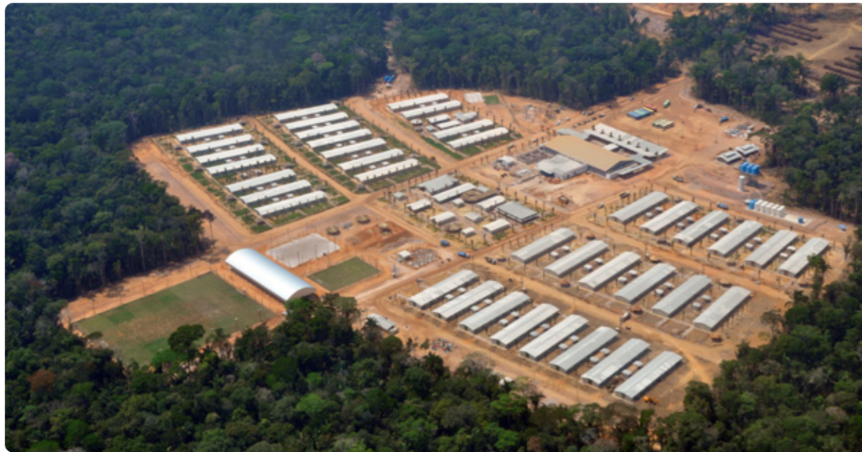
Reflecting the high standard that the consortium wished to imprint on the project, the living quarters (at the top, on the right bank; below, on the left bank) were air-conditioned and accommodated a maximum of eight workers per unit. In addition, women stayed in exclusive accommodation, reinforcing a safer and more inclusive environment.
