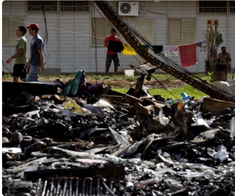
The fire led to one of the largest workforce demobilization operations ever carried out in a Brazilian construction project
