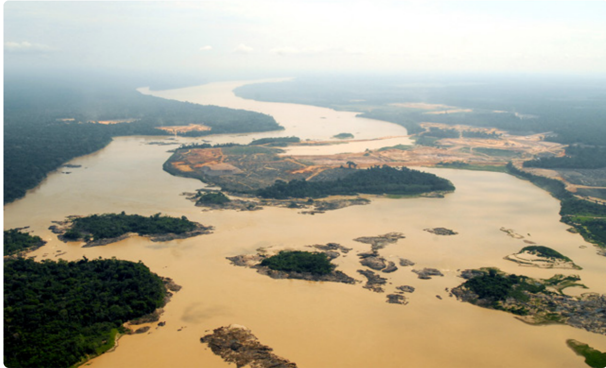
Aerial view of the Madeira River during the construction of the plant.
