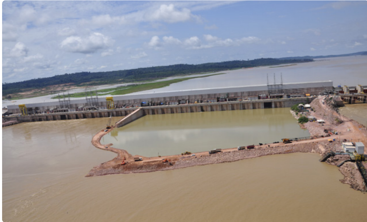
Removal of the cofferdams and the beginning of the water flow
