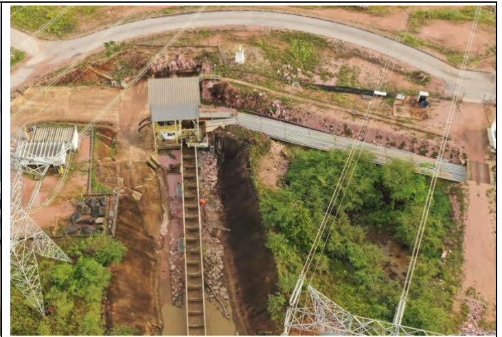
Photo 105: Aerial view of one of two fish passage facilities, with approach channel, screening building with elevators and holding basins, and pipes that supply pumped water (photo provided by ESBR)
