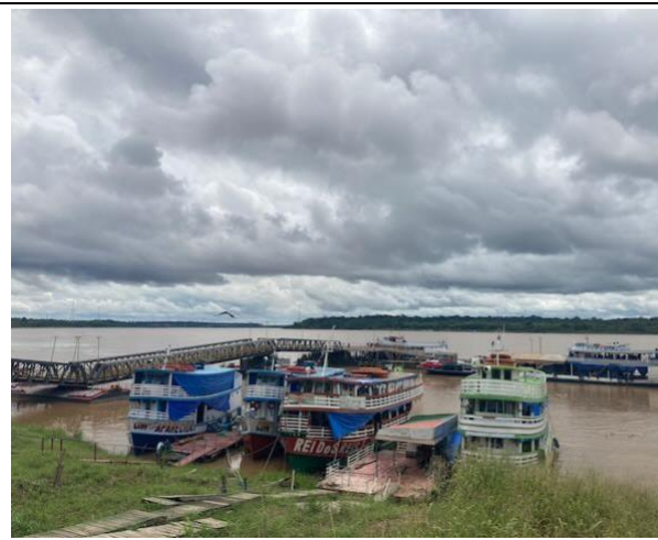
Photo 104: Porto Velho port with Santo Antonio dam in background
