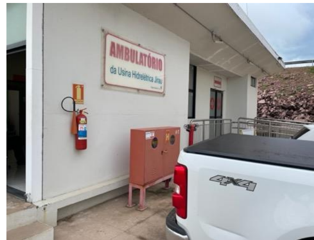
Photo 40: First aid clinic inside the powerplant
