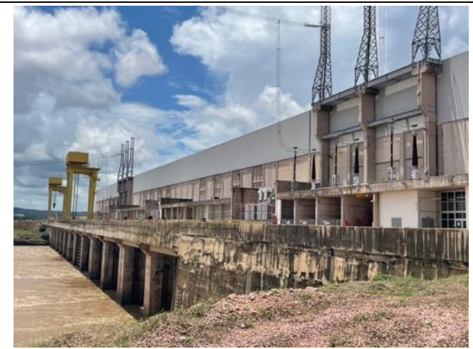
Photo 33: Left bank powerhouse from downstream
