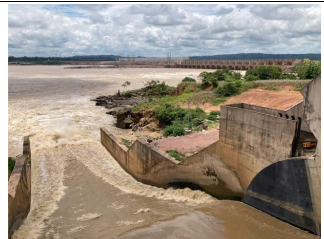
Photo 39: Log spillway with main spillway and right bank powerhouse in background
