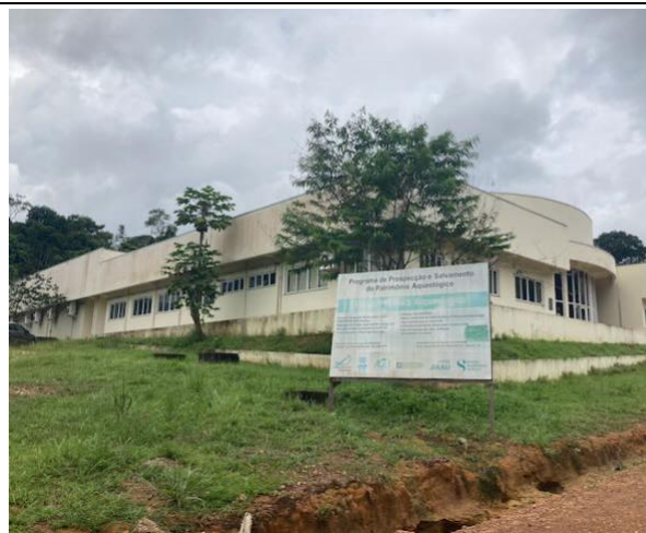
Photo 95: Archaeology building at UNIR - Universidade Federal de Rondônia - sponsored by Jirau HPP
