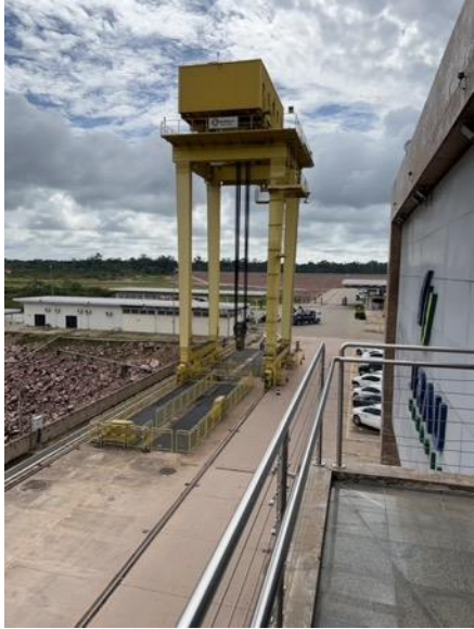
Photo 43: Downstream stop-log crane
