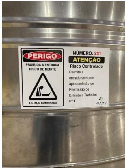
Photo 56: Confined space warning label
