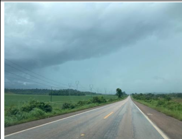
Photo 94: 3 parallel 500 kV transmission lines from Jirau HPP to Porto Velho substation along BR-364 highway
