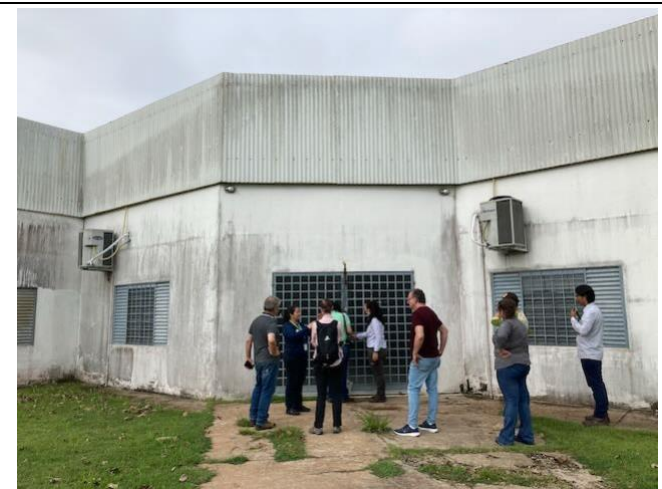
Photo 81: Disused cultural centre in Nova Mutum Paraná
