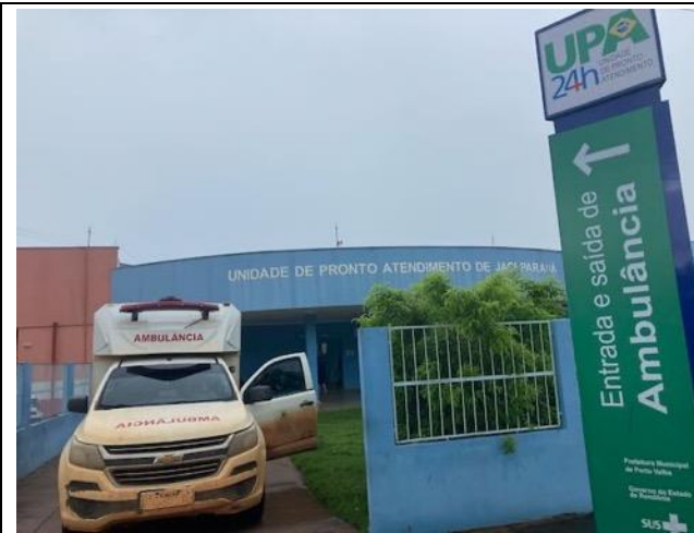
Photo 91: Health center in Jaci-Paraná, with contributions from Jirau and Santo Antonio HPPs
